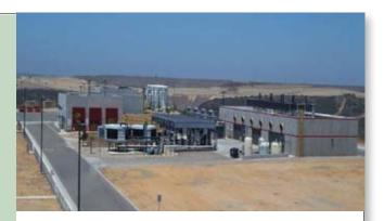
MCAS Miramar is generating nearly half of its power from this landfill gas plant, which converts methane into on-site energy. Credit: MCAS Miramar
