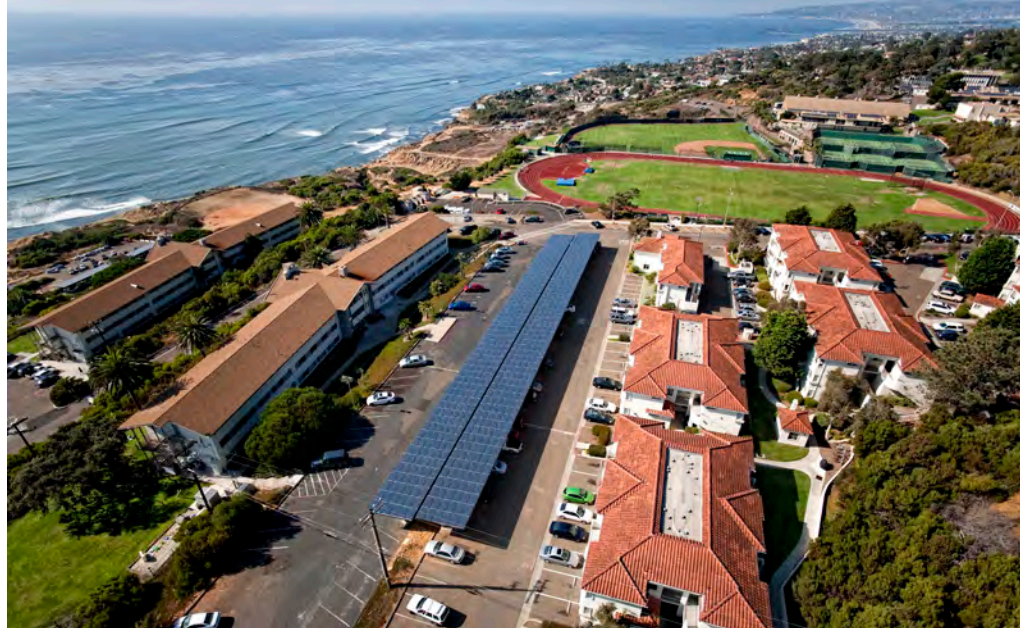
In 2011, Point Loma Nazarene University in San Diego had solar photovoltaic panels installed on top of this covered parking structure. San Diego is the leading solar city in California.
